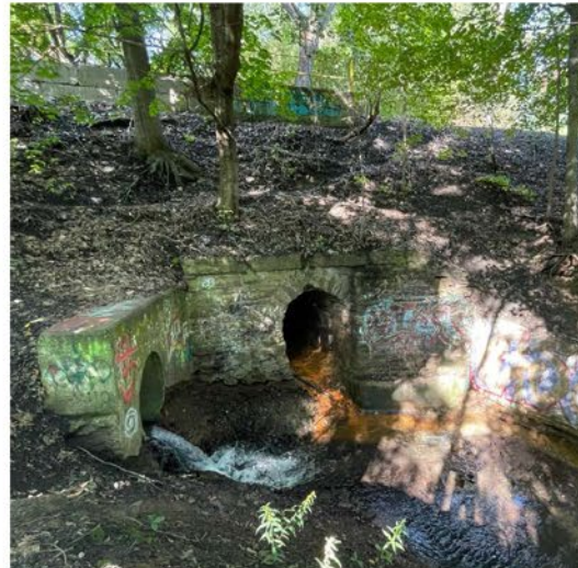
Storm water outfalls within park
