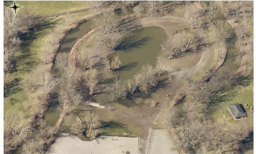
Flooding near existing dog park (2015, Monroe County GIS, Pictometry)
