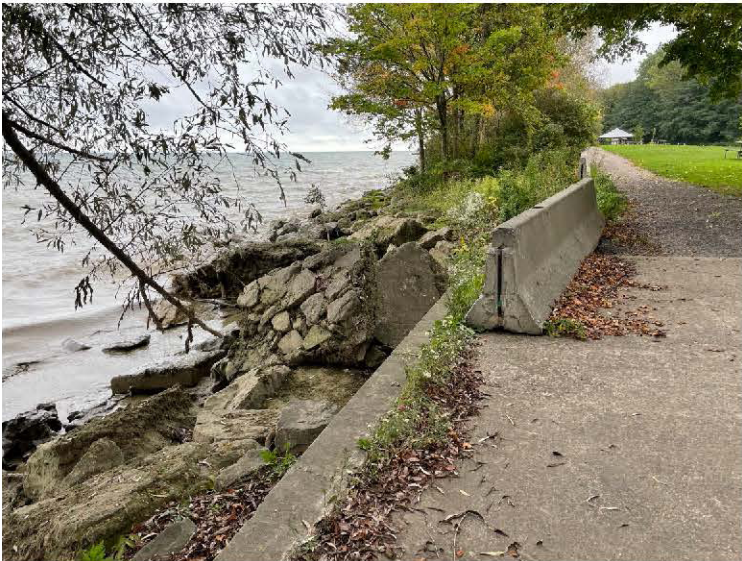
Lake front walkway and pavement undermining from wave action
