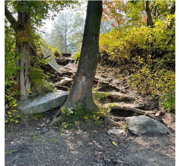
Poor access & erosion
